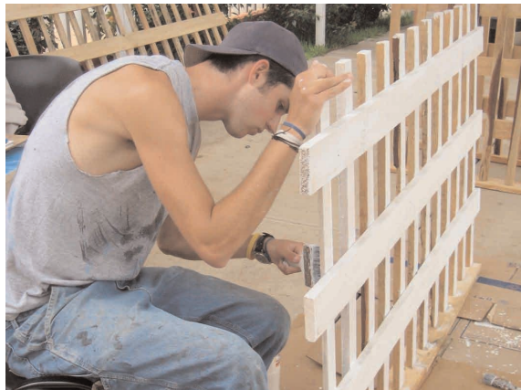
Mikey finishes up painting before using the drill.
